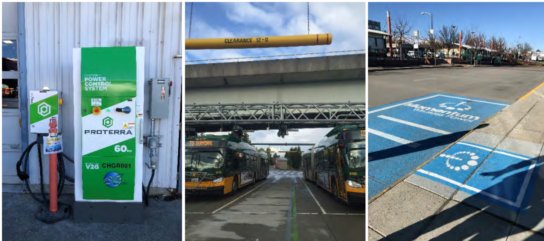
Figure 10-14 BEB Charging Methods
